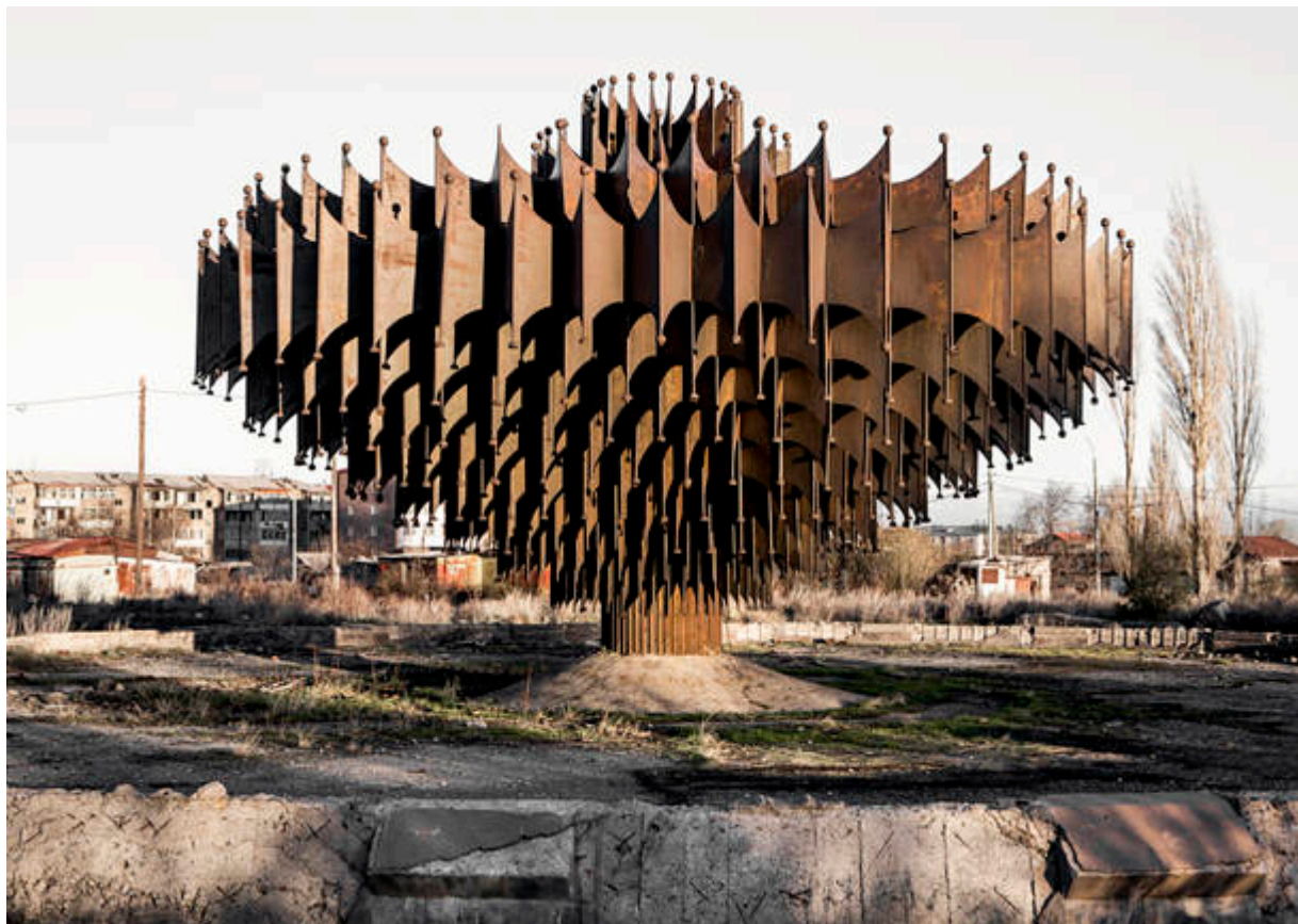
The iron fountain originally built in the area of the Polytechnic University of Gyumri by Arthur Tarkhanyan, 1982. The fountain is still standing after a strong earthquake in 1988 destroyed a big part of the city. Gyumri, Armenia.
